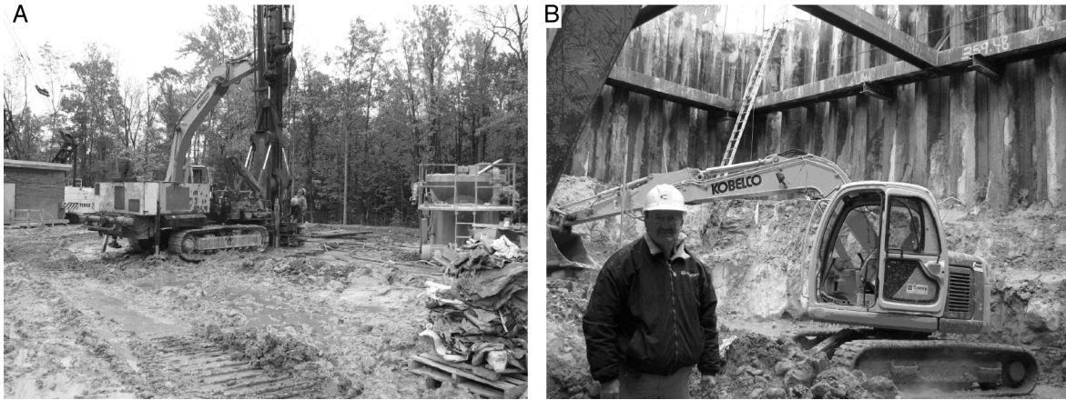
FIGURE 11 —Case History #3 photographs. A) Construction of hold-down anchors. B) Inside excavation.
