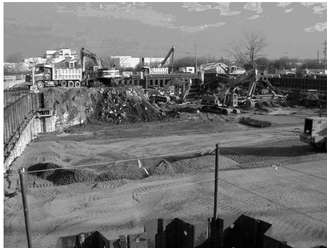
FIGURE 10 —Excavation photograph of Case History #2
